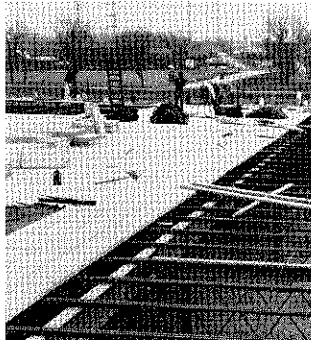
Perlite slabs are light and easy to erect; combine roof deck and insulation in one unit.
