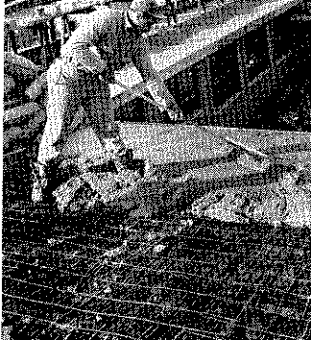
poured-in-place roof deck is light, insulating, fireproof. Screeds smooth for roofing.
