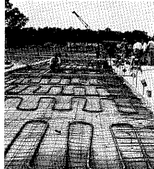
insulating slab of perlite concrete under radiant piping cuts heat loss to ground.
