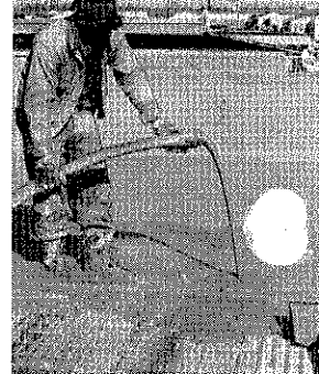
pumped-in-place roofs and sprayed-in-place walls can reduce costs.
